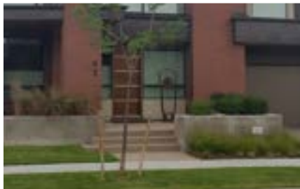
Integrate steps and site walls to create interesting site elements. Return steps to a site wall where possible.
